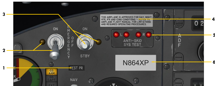
EMERGENCY BATTERY SWITCHES (APU) AND ANTI-SKID LIGHTS Figure 4-15
